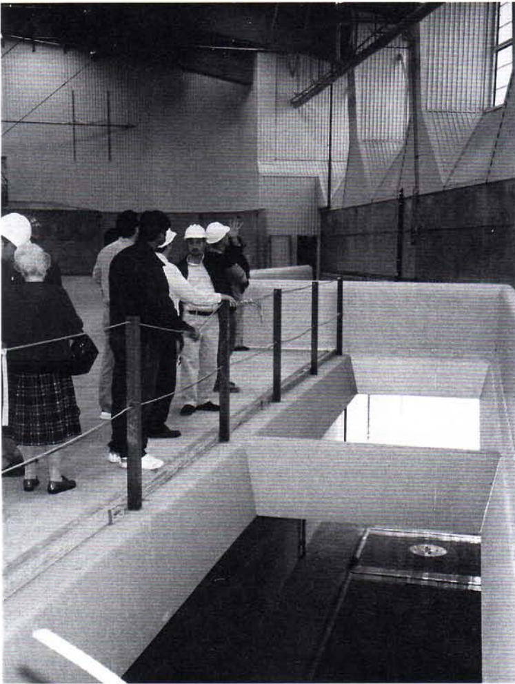
With a permitted capacity of 4,000 tons/day, and a six-day weekly capacity of 24,000 tons, residual waste will be pushed into containers via these loading drops. The containers will then be trucked to a nearby intermodal facility for rail transport to the Districts-owned and fully permitted Mesquite Regional Landfill in Imperial County, about 200 miles from Los Angeles.
